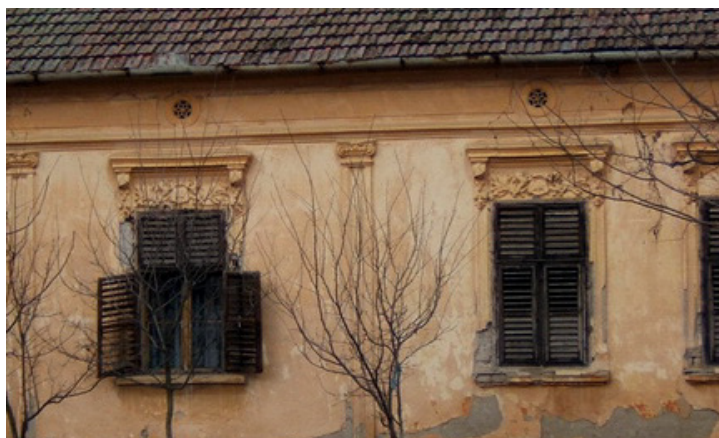
Figure 2 An example of a ventilation opening, above a window, on an old Vojvodina house
